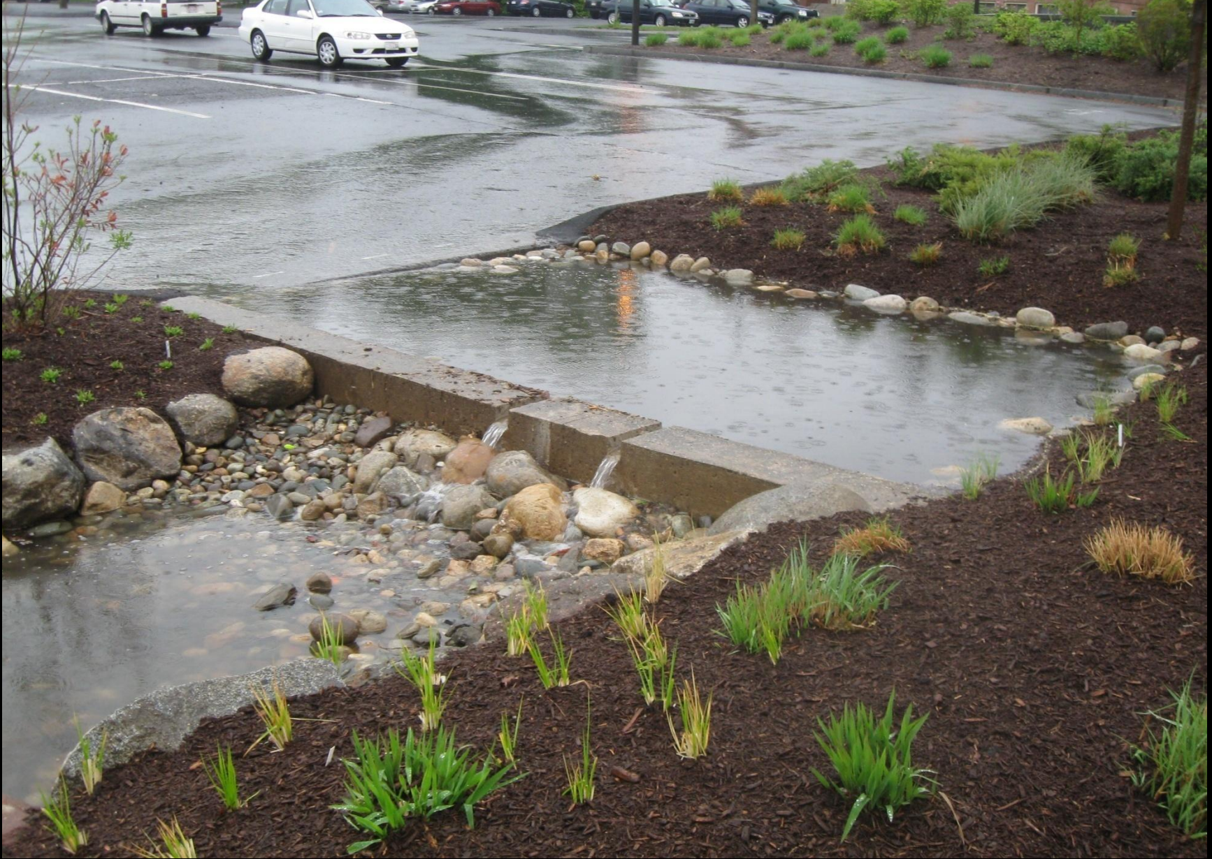
Raingarden: Planted with native species for water quality renovation and biodiversity value
